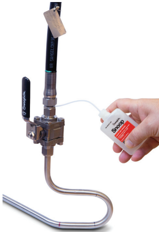
Figure 7-3 Snoop leak test.
